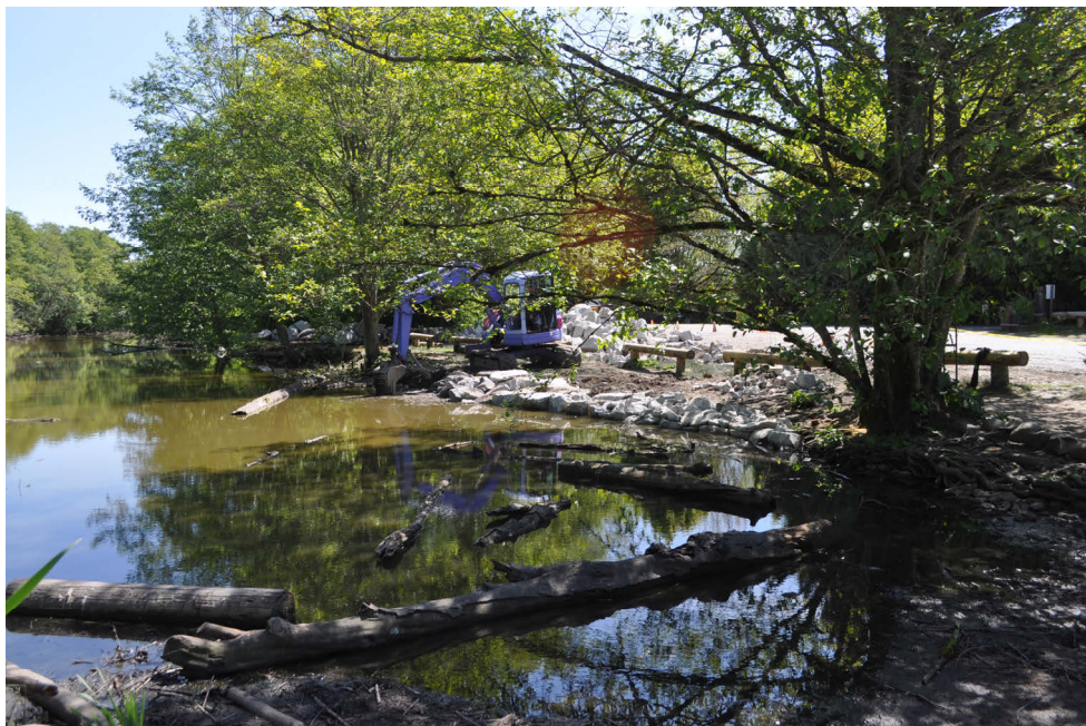
Excavator placing rock along Robertson Slough at the parking lot.
